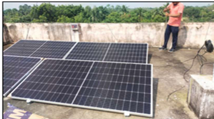
Solar panel Installation in Government school Kundrathur, Smile Foundation
