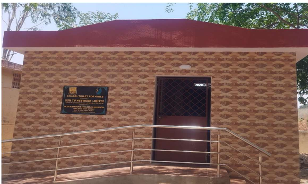
Krishnagiri – Toilet facilities – SISO
