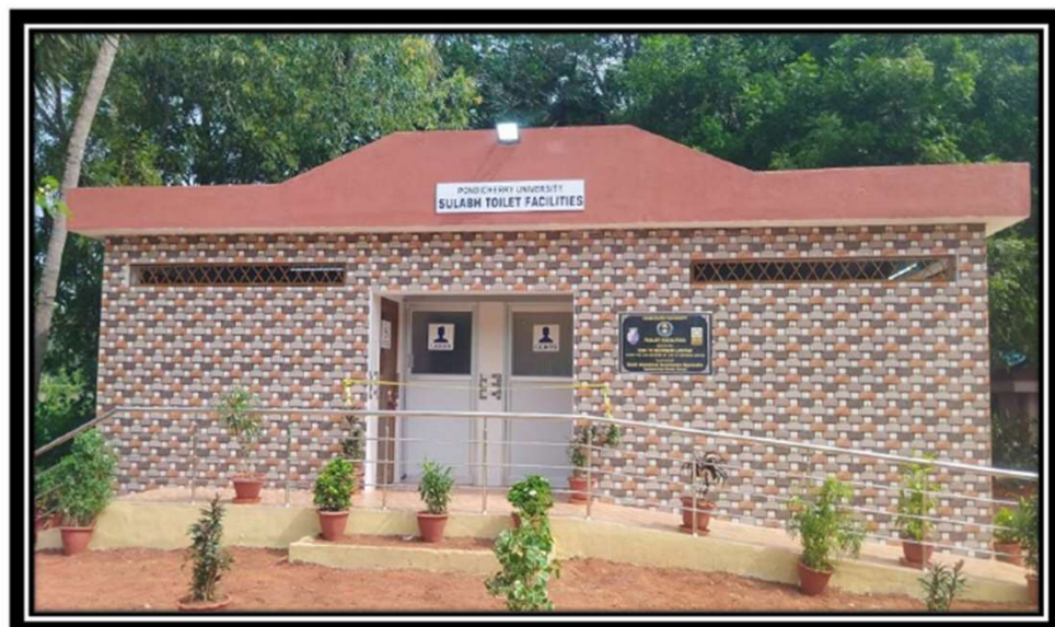
Pondicherry University – Toilet facilities – SISO
